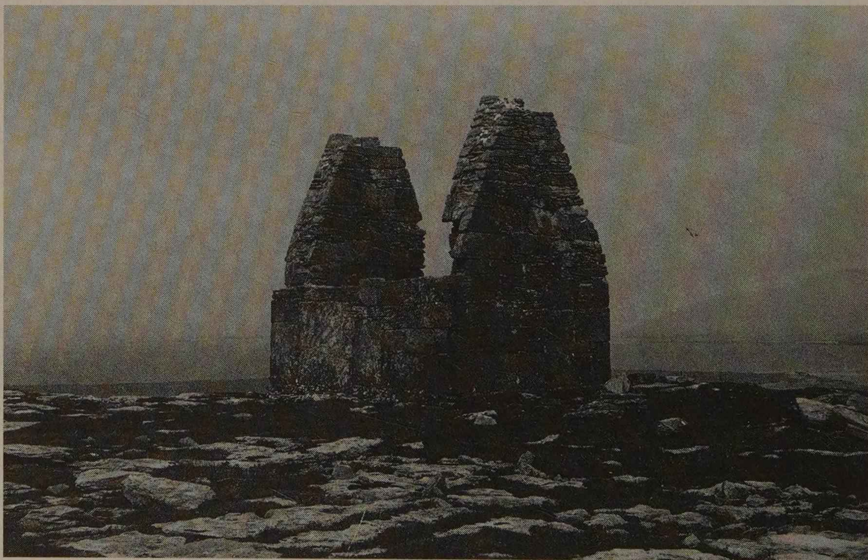
51 Tempall Benén (Church of St Benignus), Aranmore (Co. Galway). This tiny but impressive little church consists of a single chamber, oblong in plan, measuring internally only 10\frac{1}{2} by 7 feet, with no division between nave and chancel, and about 15 feet high. Its orientation, almost exactly north and south, is unique. The side-walls contain some very large stones. The site is splendidly chosen, for despite its small size, this hill-top church is a land-mark visible far out in Galway Bay.
