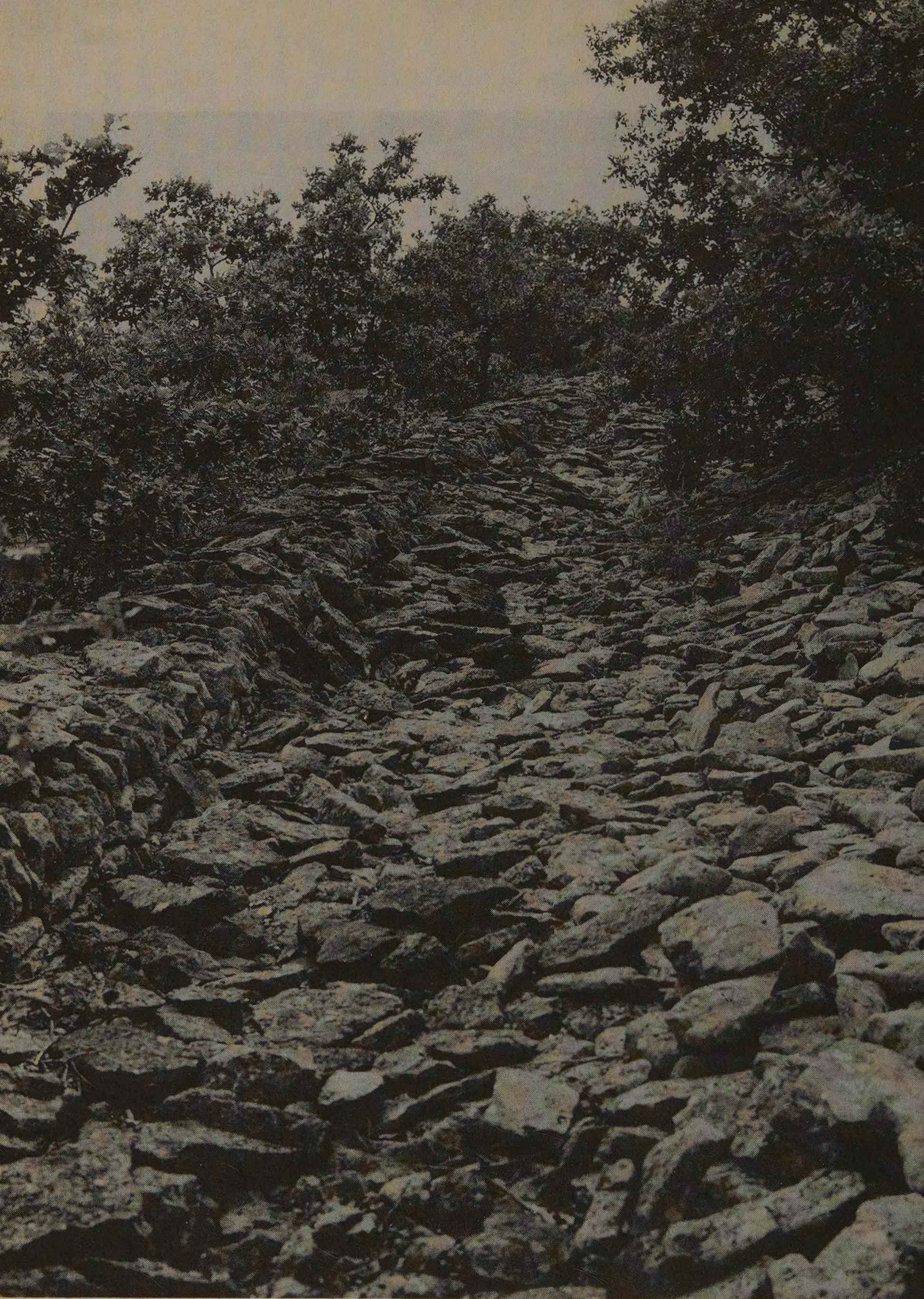
2 Pre-Roman road between Saignon and Sivergues, on the high plateau of Claparedes (Vaucluse). The road is stone-paved and the kerb on the left is clearly preserved.
