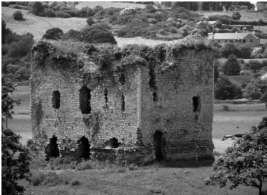
36 The donjon at Grenan. The toilet chute from the big first-floor room is visible in the short wall. The ground-floor entrance to the tower (with a small chapel above it at first-floor level) was at the opposite end, facing the probable site of the hall.
