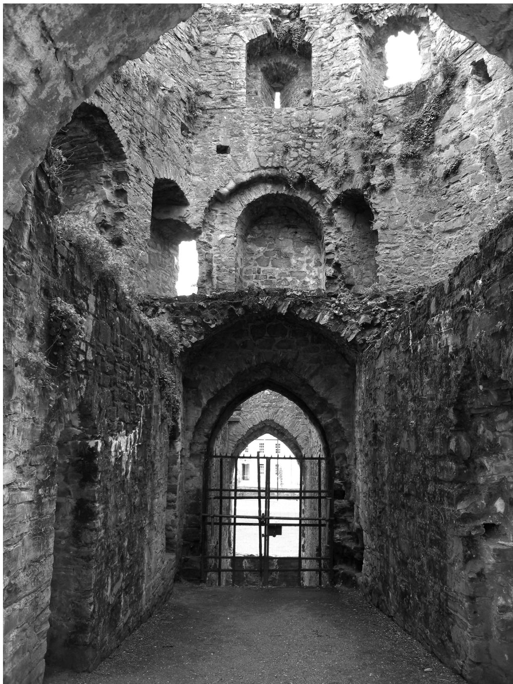
48 The interior of the Dublin Gate of Trim Castle, showing the round arch at first-floor level, and a similar arch in the original, 1170s, part of the donjon ( opposite ).
