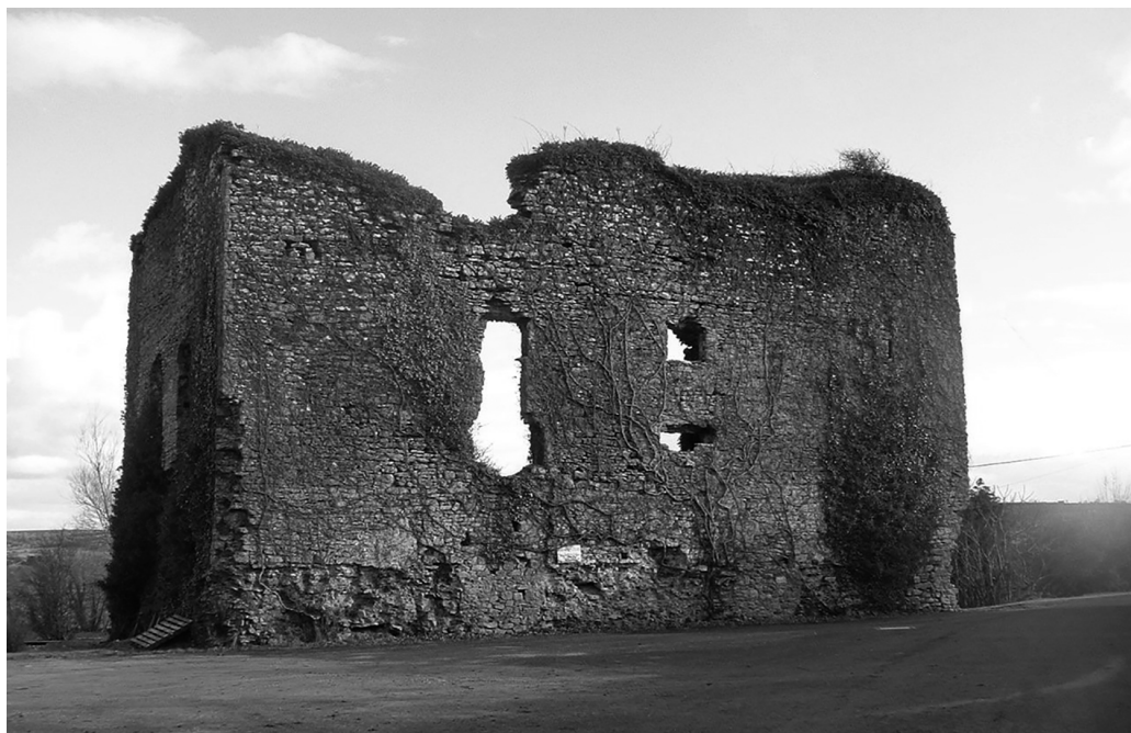
33 The donjon at Ballyderown. The two large windows are visible on the left-hand side. The walling on the far right-hand side belongs to a late medieval toilet turret, making the tower look slightly longer than it was originally.
