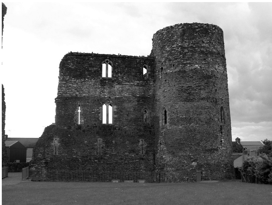
68 The exterior of Ferns Castle. The surviving turret on the right-hand side contains the vaulted chapel.
