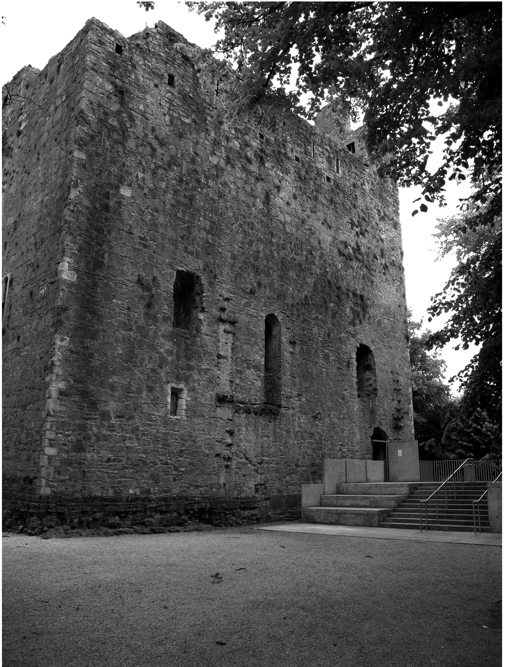
25 The donjon at Maynooth. The original entrance at first-floor level is on the far right-hand side. The door in the middle of the wall at that level connected the hall to the chapel in the (now-lost) fore-building.
