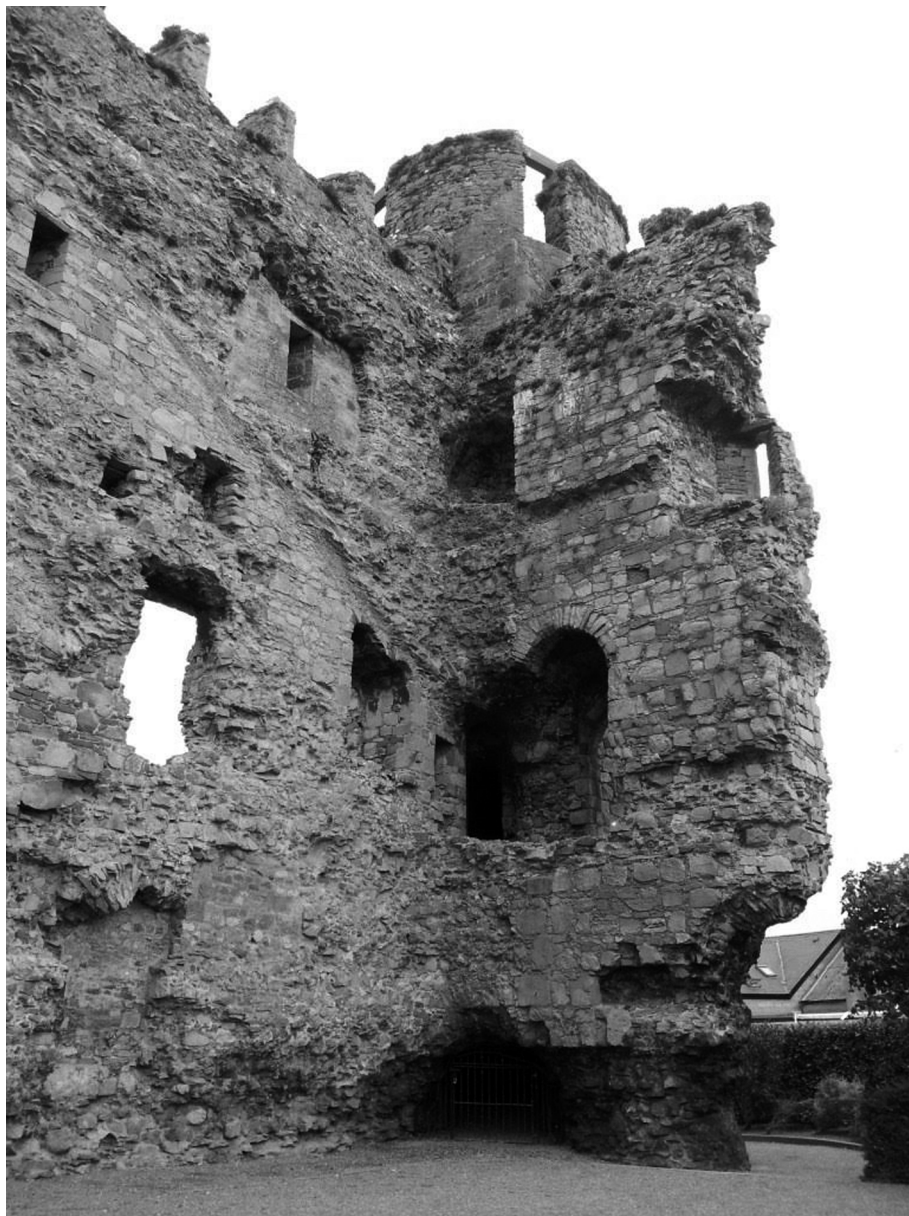
64 Carlow donjon interior. The truncated north wall with the entrance at first-floor level ( above ); the long west wall, with the ascending scar of the now-destroyed vaulted stairs-passage ( opposite top ); the south end of the west wall, with traces of the vaulted stairs-passage which descended into the basement, and the truncated south wall ( opposite bottom ).
