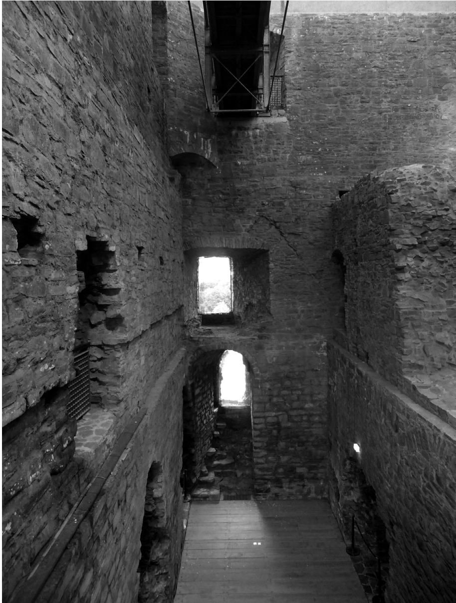
23 The original first-floor chamber in Trim donjon, viewed from inside the original roof-space, with the cross-wall on the right-hand side. Note the outline of the original pitched roof on the opposite wall, cut through by a later window.
