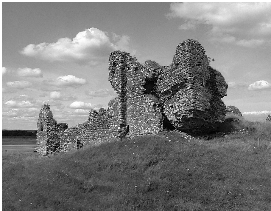
40 The collapsed corner at one end of Clonmacnoise Castle, showing the pilasters at the narrow end of the donjon; the remainder of the donjon extended to the right.
