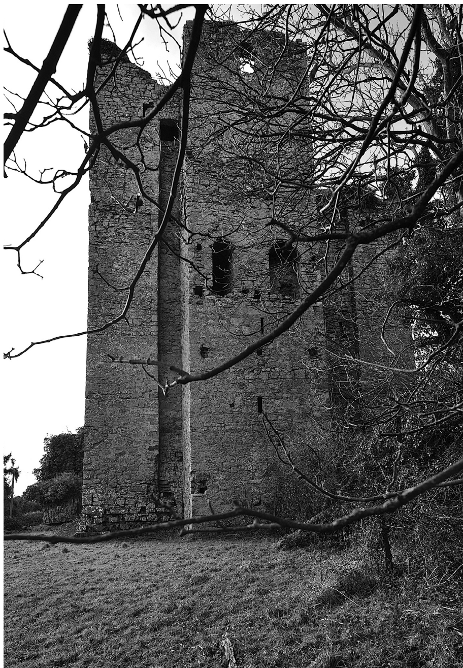
42 The donjon at Coonagh, showing the projecting turret. The arch on the right opens into the turret, and that on left is a recess. There are very slight traces of scarring from the original timber roof above the two features. There are signs on the mortar plaster that the fore-building wrapped around the turret on the left-hand side. An original window at ground-floor level in the turret suggests that the fore-building was partly open-framed.
