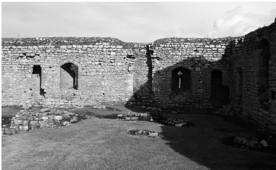
87 Small chambers, probably lodgings, inside Ballymoon Castle. The doorways lead to toilets; the chutes of toilets drop down within the wall thickness from the unbuilt upper floor, suggesting that floor was to mirror the one which survives in part today.
