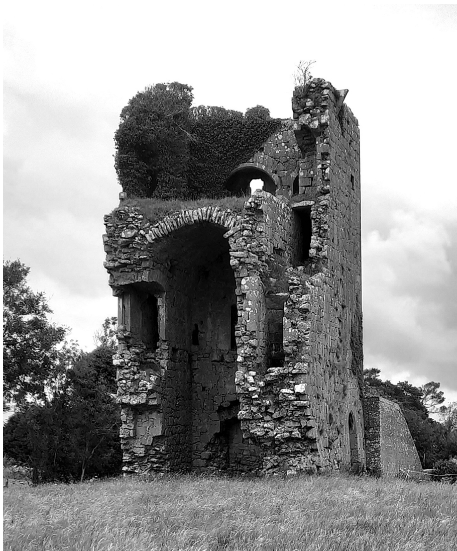
89 The tower-house in Garbally (Galway) was extant in 1504, so it dates from the fifteenth century; it is probably post-1450 to judge by its architectural detailing. Note the large room at the top, above the vault.
