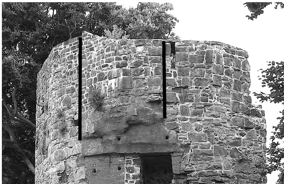
54 The two black lines mark the edges of the buttress which projected slightly at the entrance at Castleknock.
