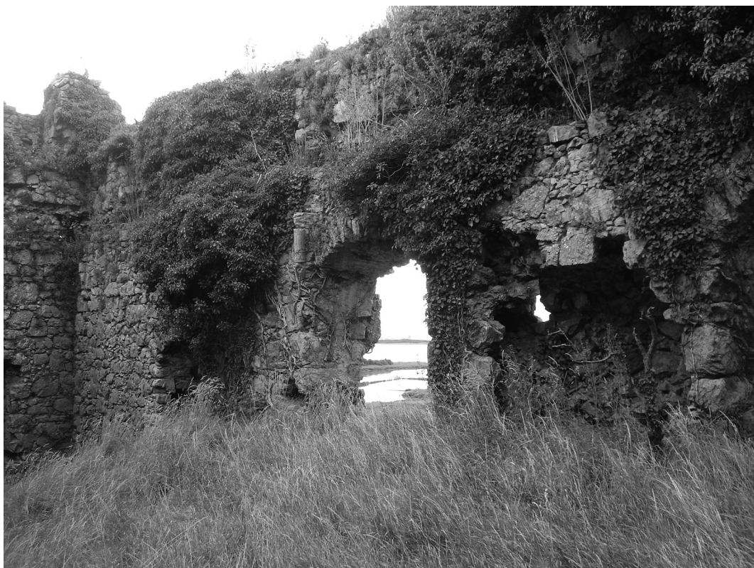
35 The interior of Tomdeeley donjon. Note the small fragment of an engaged shaft to the left of the doorway. It is unlikely that there was an arch above this, so the spatial division might have been effected by articulation on each side wall, with a less permanent screen between.
