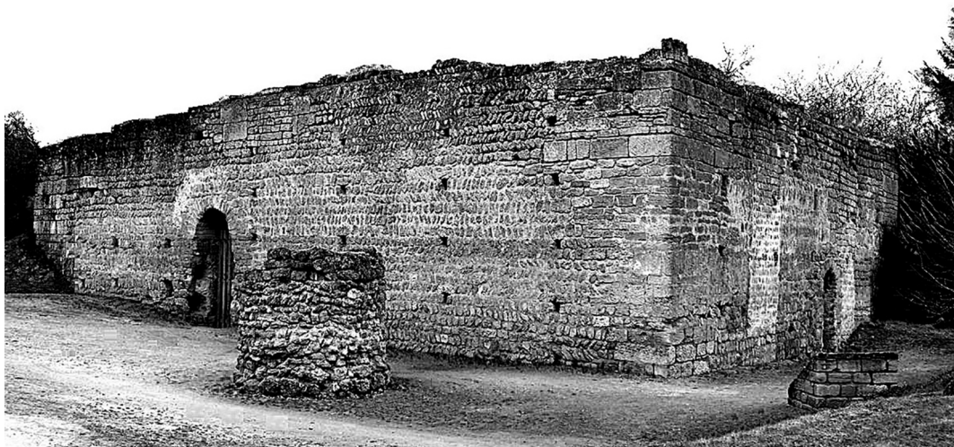
13 The aula/turris of Doué-la-Fontaine. The interior was divided into two spaces of unequal size by a latitudinal wall with a connecting doorway. The doorway on the left leads into the larger space, originally heated by a central hearth; the small doorway on the right leads into the narrower space, heated by a wall fireplace.
