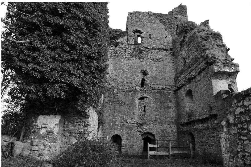
41 The interior of Coonagh donjon. The two doorways at different floor levels in the end wall are original. As with Maynooth (see Fig. 27), the fabric does not allow an easy reconstruction of the original roofing.
