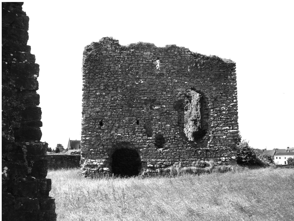
32 The donjon at Glanworth. The original entrance is at first-floor level on the right-hand side. The small slit window at the top of the wall was originally just under the roof.
