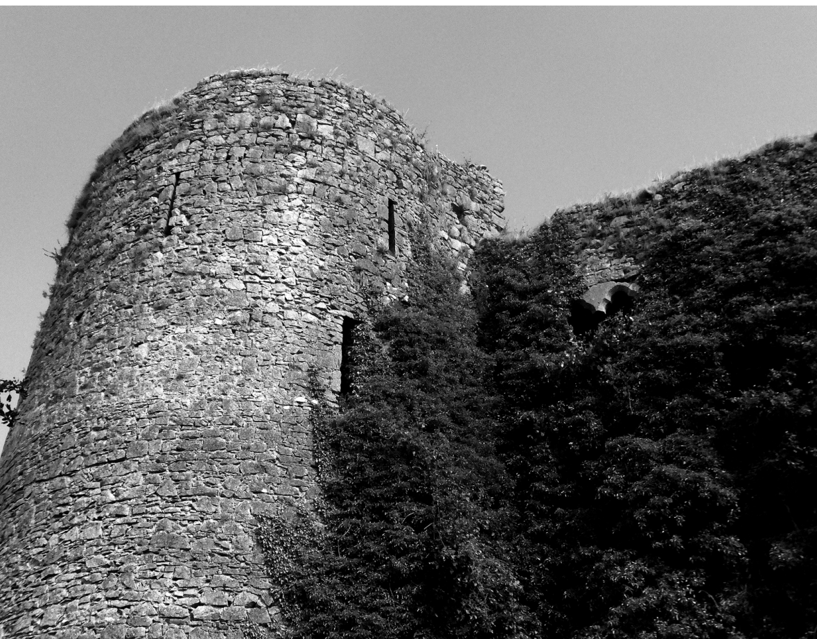
65 Part of the exterior of Lea Castle, showing the top of the only intact corner turret and (partly hidden by vegetation) the twin-light window to which all writers on the castle have drawn attention for dating purposes. One can see a slight change in the fabric of the turret, corresponding to the level at which the tower was extended upwards by a single storey in the third quarter of the thirteenth century.
