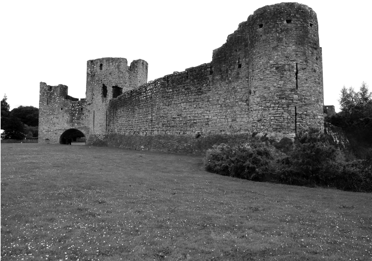
47 The Dublin Gate and adjacent curtain wall at Trim Castle. Slight changes in fabric and/or alignment of the curtain wall indicate that the barbicaned gate-tower (with adjacent short stretches of walling) was built first, followed by the tower to the south (on the right-hand side in the photograph), followed by the curtain wall between them.
