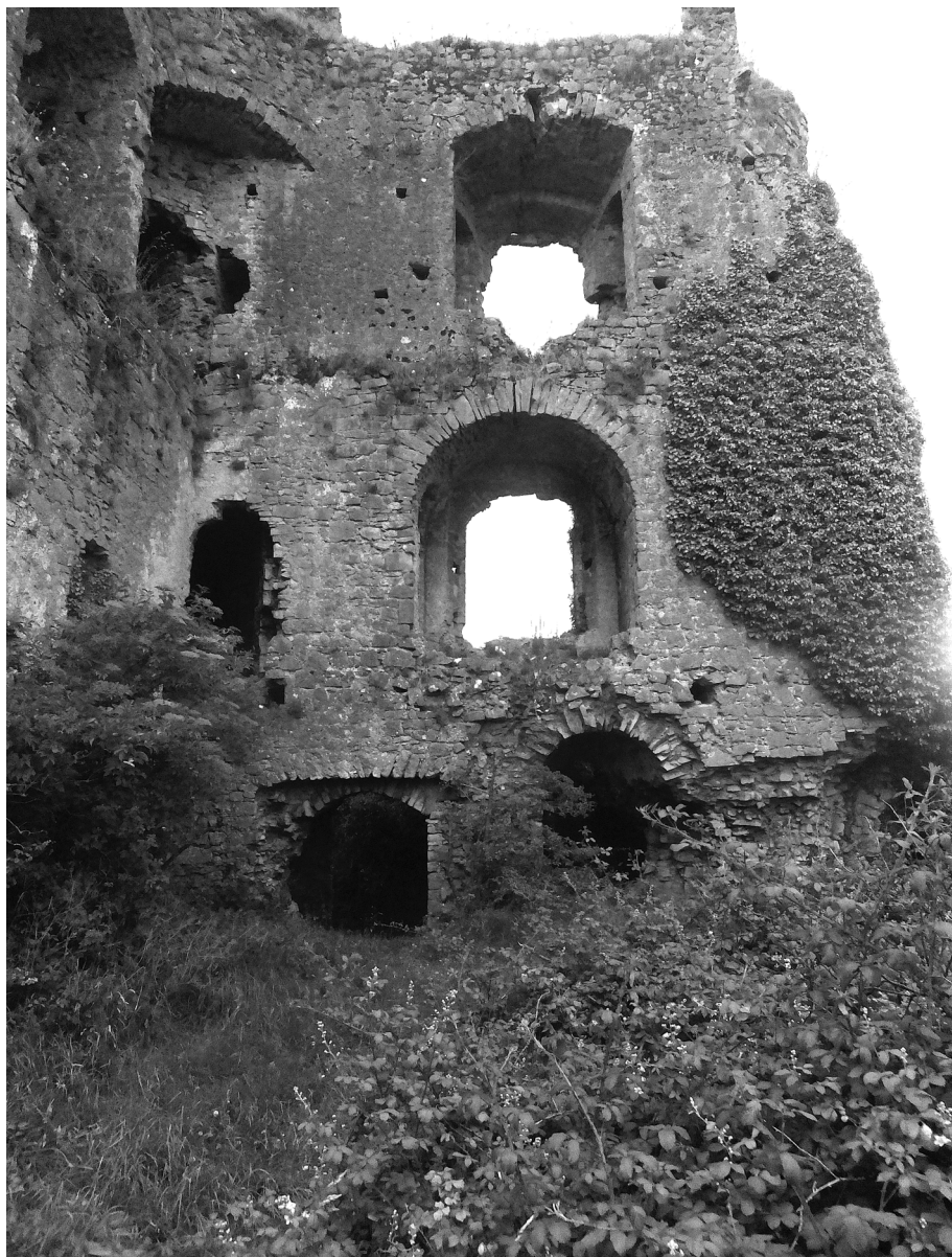
66 The interior of the donjon at Lea, photographed from first-floor level. The chapel recess is visible in the end wall, above the original first-floor entrance with its round-arched doorway.
