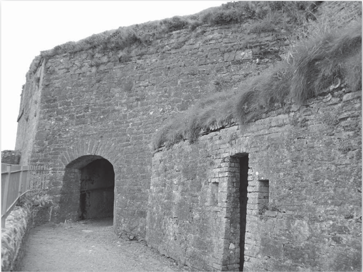
This close-up of Duncannon Fort shows clearly how the advent of gunpowder weapons had begun to affect fortress design. Walls were now thicker and more squat to absorb the impact of enemy shot whilst they were also often angled to deflect incoming cannon balls. (Kieran Laffan)
