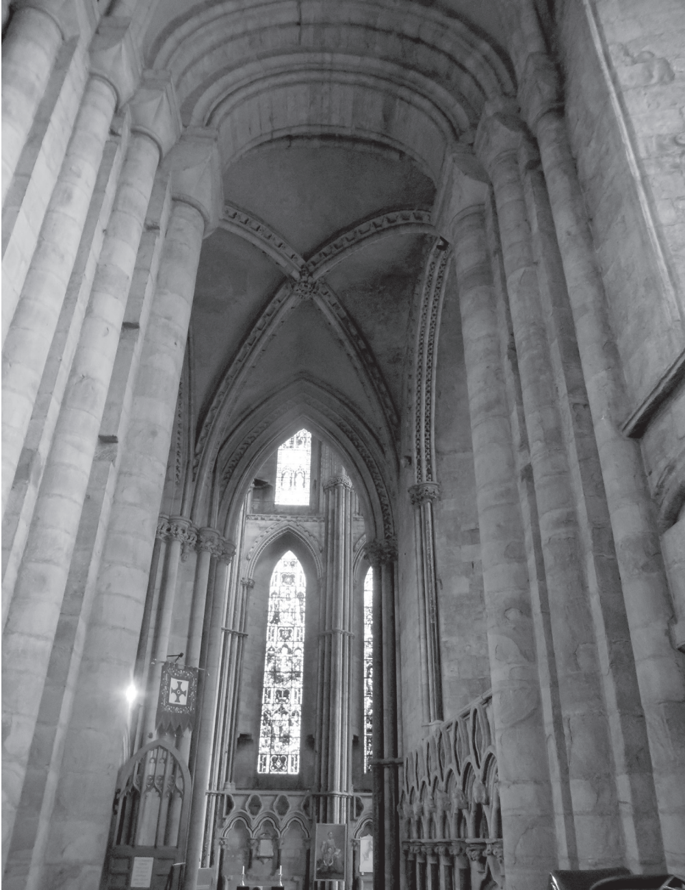
FIG. 7.6 SOUTH CHOIR AMBULATORY OF DURHAM CATHEDRAL LOOKING EAST, SHOWING CUTTING AWAY ON PIER ON NORTH SIDE AND AT CORRESPONDING LEVELS ON PILASTER ON SOUTH SIDE:
