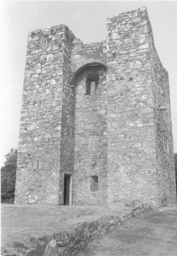
Figure 128 Audley's castle, Co. Down: the door of the tower-house protected by the two turrets and a machicolation arch
