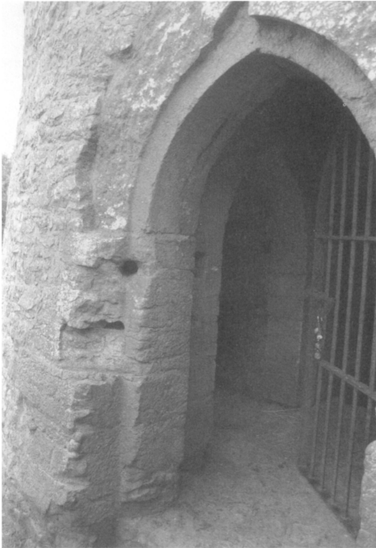
Figure 131 Ballynahow castle: the tower-house door with the emplacement for a 'yett'
